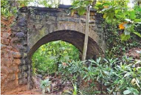
One of the remaining arch-culverts on the Kelani Valley line
