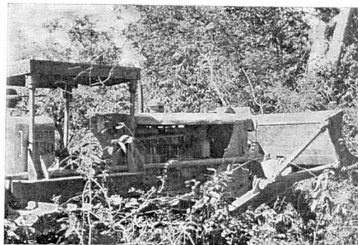
Typical jungle in which the Batticaloa Airstrip was built. D8 Tractor, supplied by the Gal-Oya Board and operated by Volunteer Plant Squadron, Ceylon Engineers, felling trees
