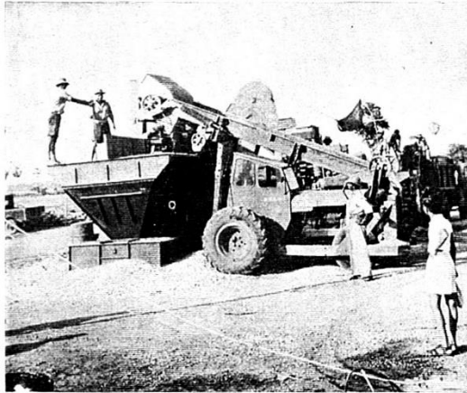
Overloader feeding Barber Green Road Laying Pre-mix Plough, supplied by P. W. D. and operated by P. W. D. crews and Army personnel
