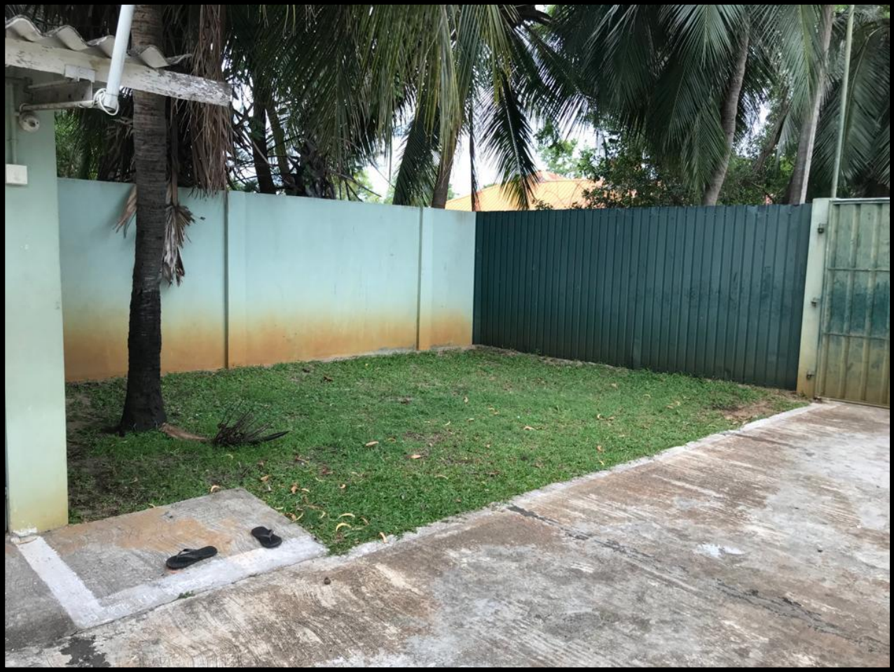
Back View of the place allocated for toilet construction
